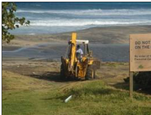
Figure 20: Public Works attempting to sand mine eroded area of Zeelandia Beach.
